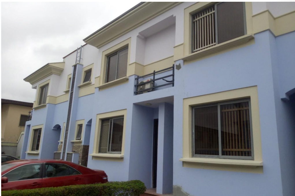
50 – ALUMINIUM WINDOWS & DOORS FOR RESIDENCE IN SURULERE.
