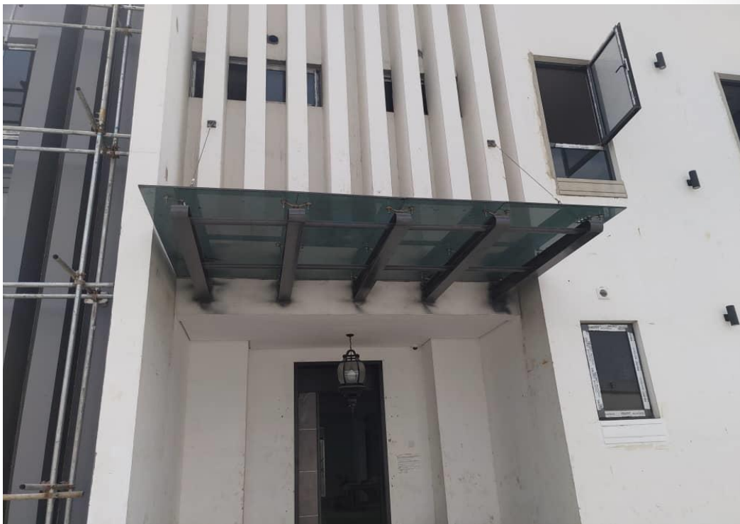
ENTRANCE CANOPY AT IKEJA, GRA.
