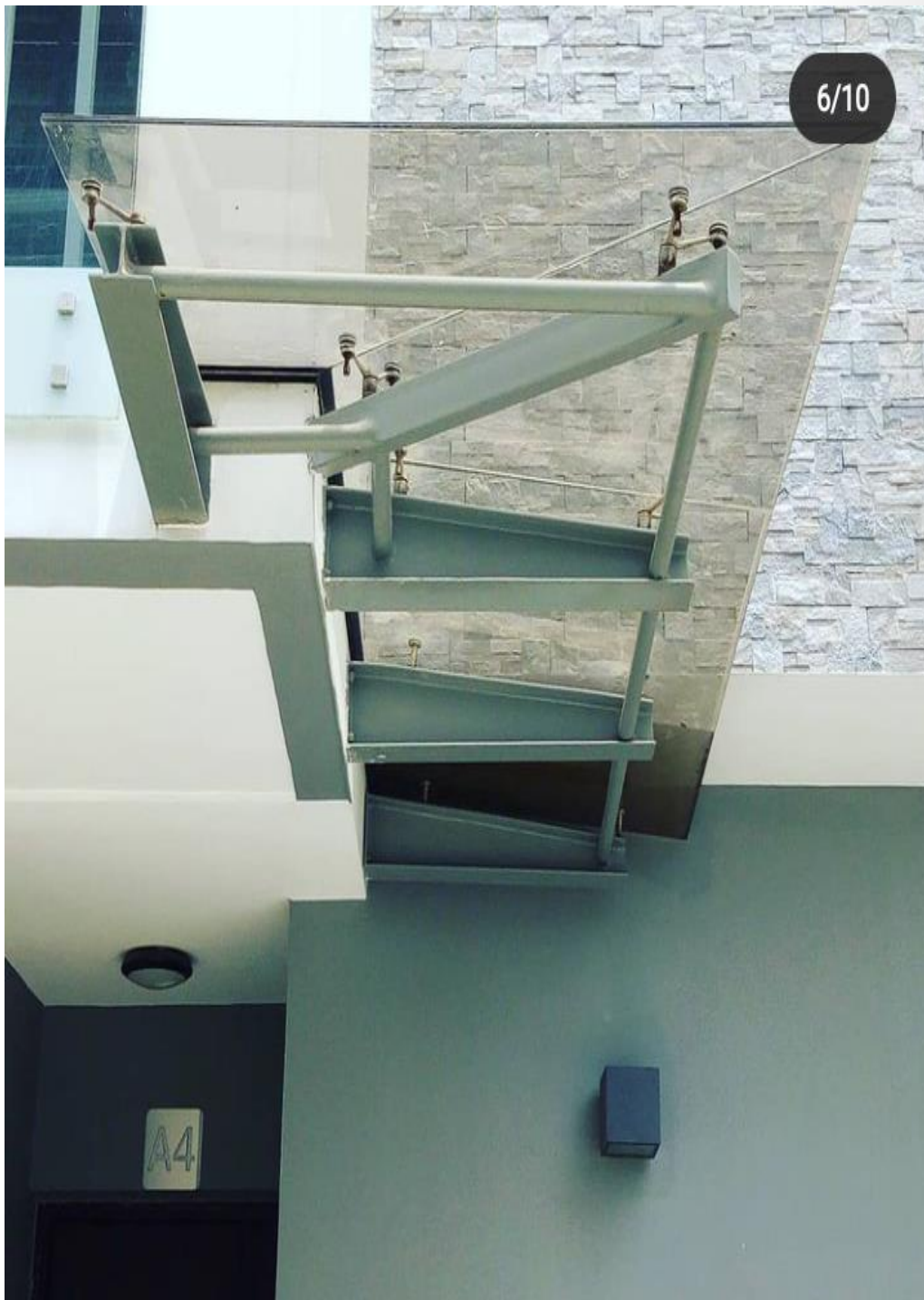
61 – LAMINATED GLASS ENTRANCE CANOPY FOR RESIDENTIAL DEVT. IN IKOYI.
