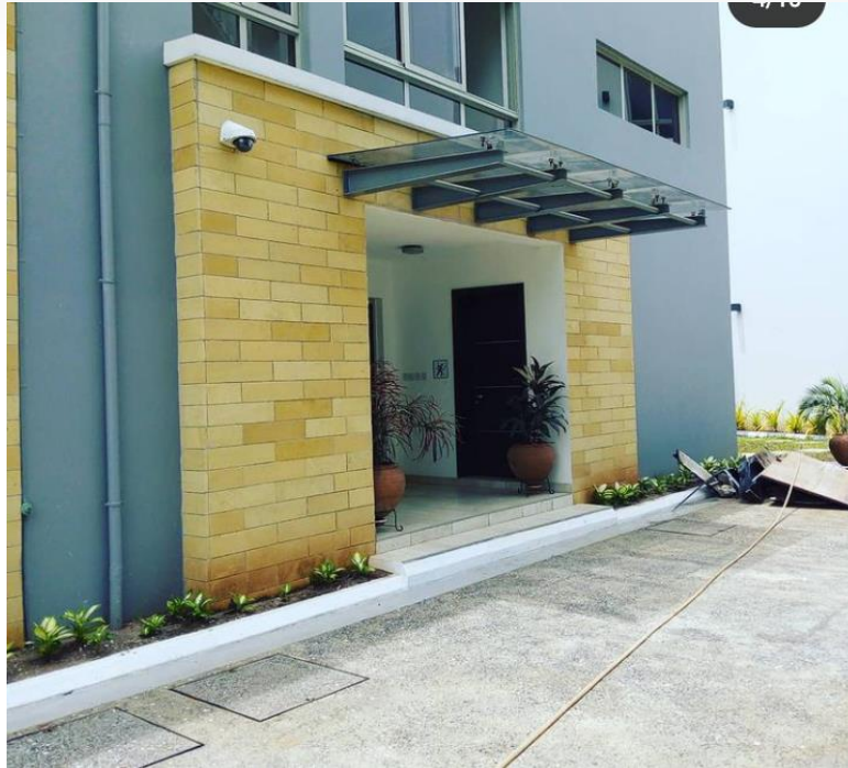
63 – LAMINATED GLASS ENTRANCE CANOPY FOR RESIDENTIAL DEVT. IN IKOYI.
