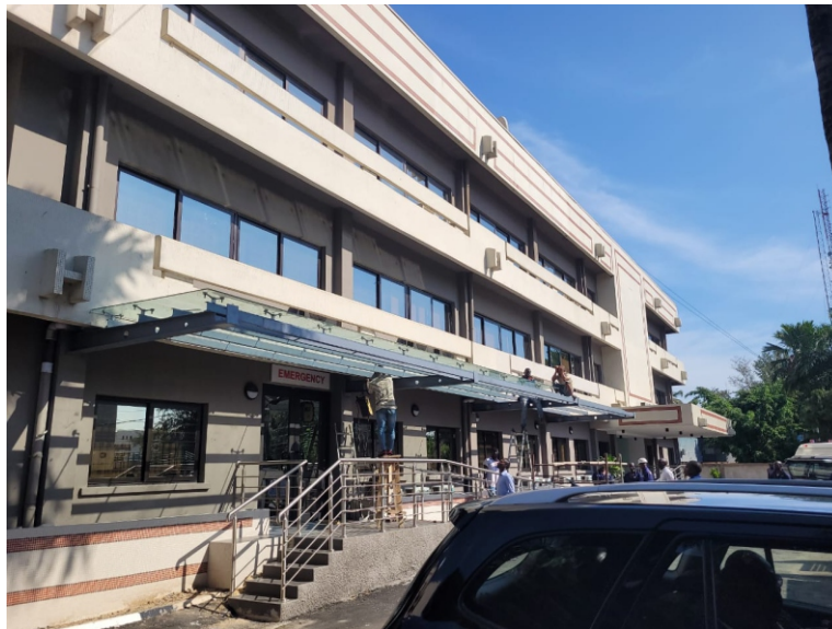
Grade 316 Stainless Steel Handrails at Lagoon Hospital, fabac close, Victoria-Island, Lagos.
