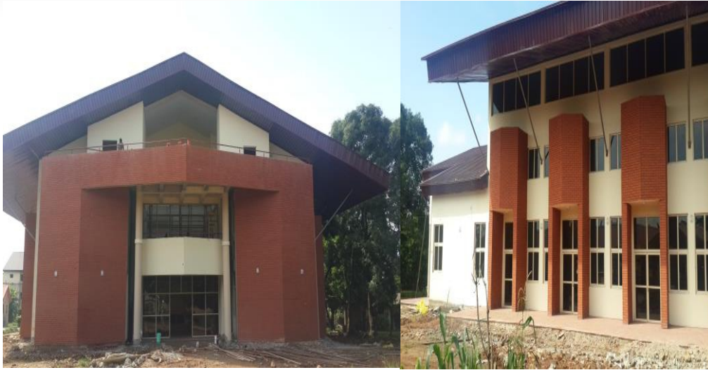
ALUMINIUM ROOFING, WINDOWS, DOORS AND CURTAIN WALLS FOR NEW AUDITORIUM BUILDING AT METHODIST TRAINING INSTITUTE, SAGAMU.
