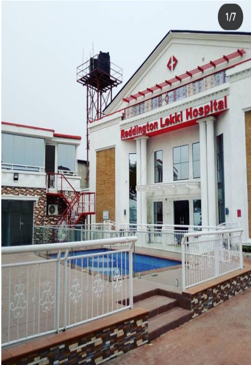
66 – FRAMELESS GLASS PARTITION AT REDDINGTON, LEKKI.
