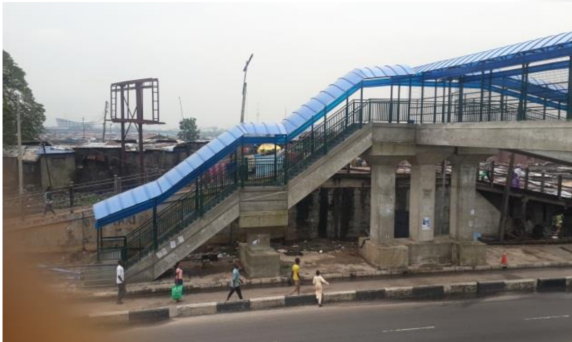
WALKWAY HANDRAILINGS; 'CLEAR VU' FENCING AND POLYCARBONATE COVERING (DANPALON) FOR PEDESTRIAN BRIDGES AT FADEYI / OTTO BUSSTOP IKORODU ROAD, LAGOS.
