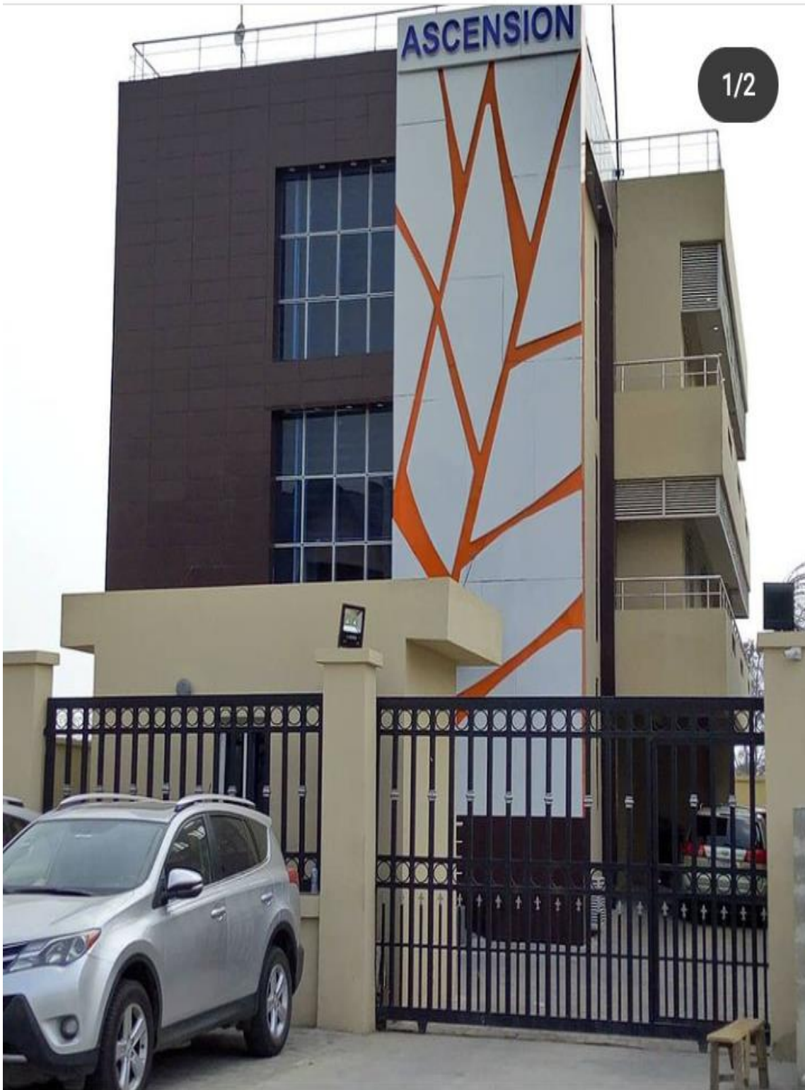
25 – ALUBOND CLADDING/ENTRANCE GLASS CANOPY IN LEKKI.
