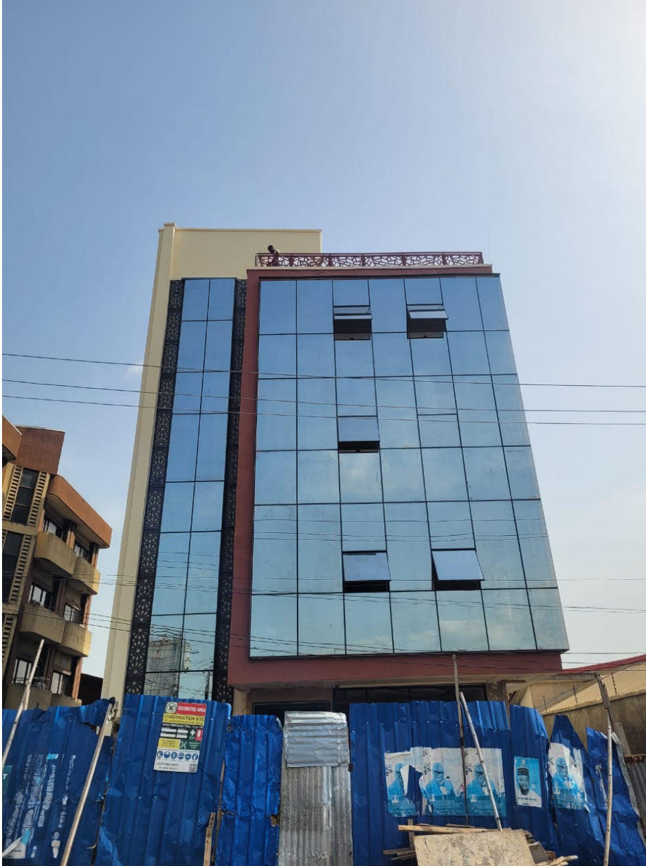
Glazed Concealed Grid Curtain walls for CONTROL SYSTEMS INT'L CO. LTD at ILUPEJU - LAGOS.
