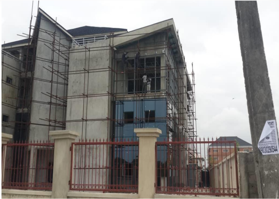
37 - DOUBLE GLAZED STRUCTURAL CURTAIN WALL WITH ALUCOBOND CLADDING.
