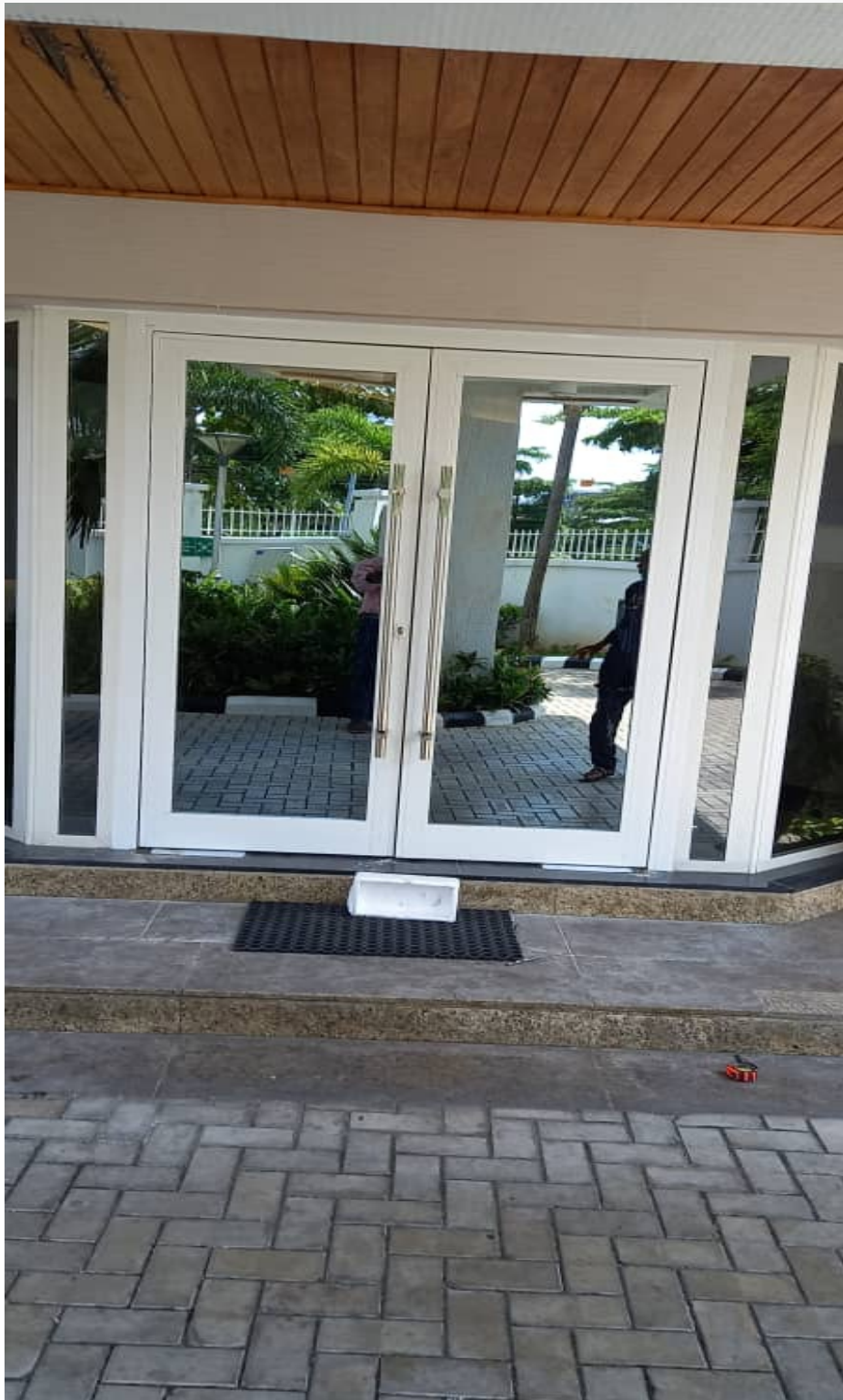
ALUMINIUM FRAMED ENTRANCE GLASS DOORS FOR SAHARA ENERGY TOWERS AT BANANA ISLAND, IKOYI, LAGOS STATE.
