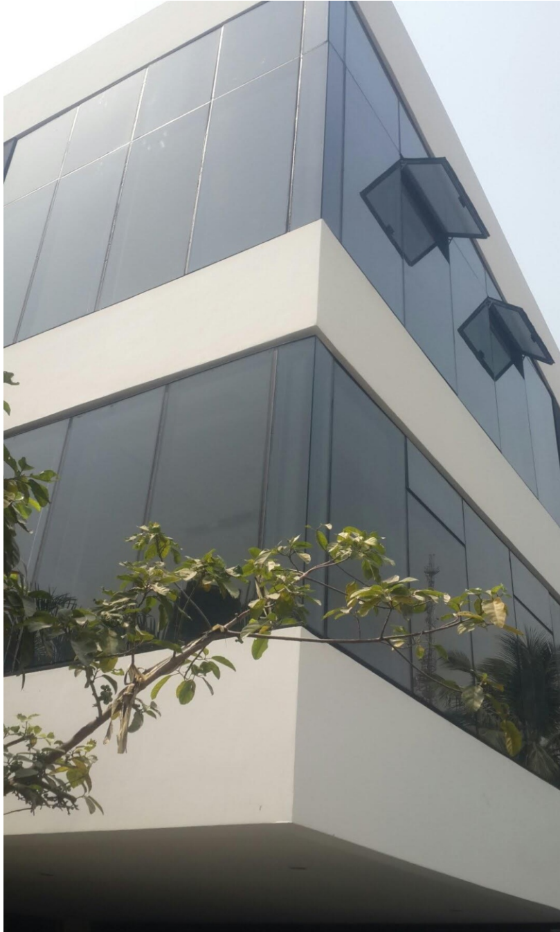
16-LAMINATED STRUCTURAL CURTAIN WALL AT TEMPLE MUSIC, VICTORIA ISLAND.
