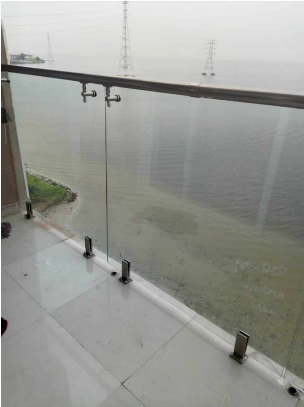
FRAMELESS CLEAR SAFETY GLASS BALUSTRADES AT LEKKI PHASE 1, LAGOS.
