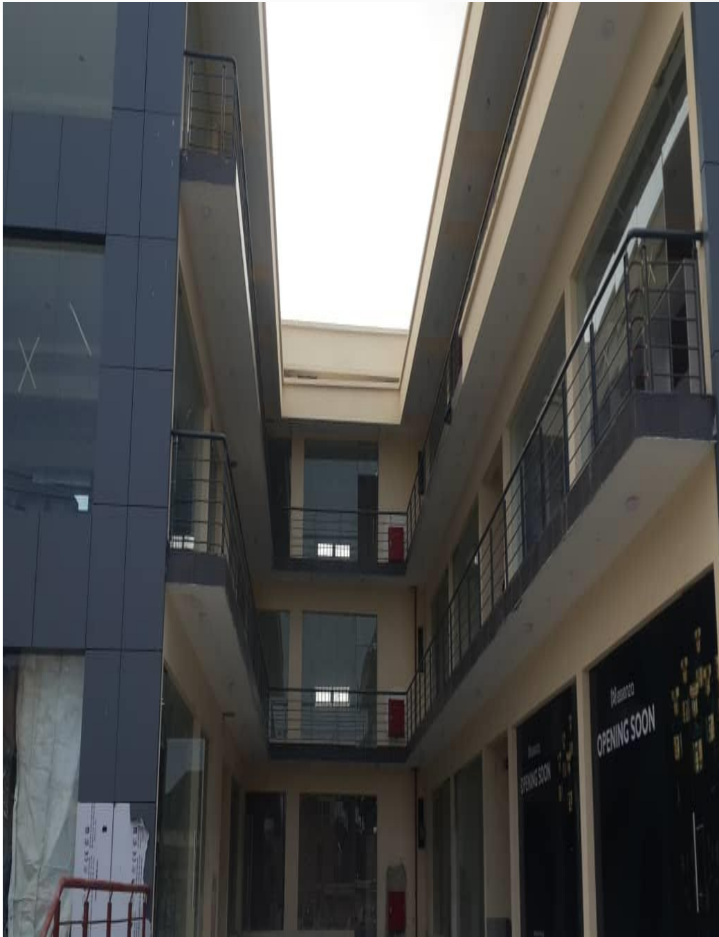
39 – FRAMELESS GLASS SHOP FRONT AT GREENVILLE SHOPPING MALL, ADMIRALTY WAY, LEKKI.
