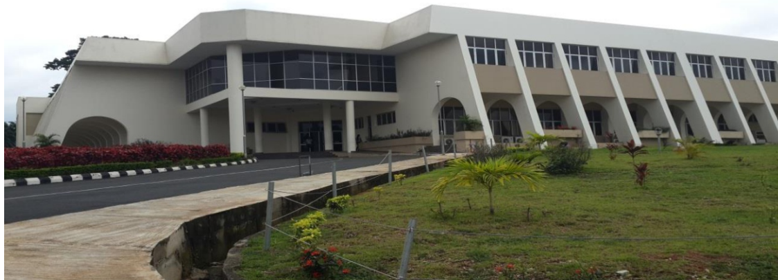
ALUMINIUM ROOFING, WINDOWS, DOORS AND CURTAIN WALLS FOR NEW INTERNATIONAL CONFERENCE CENTRE UNIVERSITY OF IBADAN.
