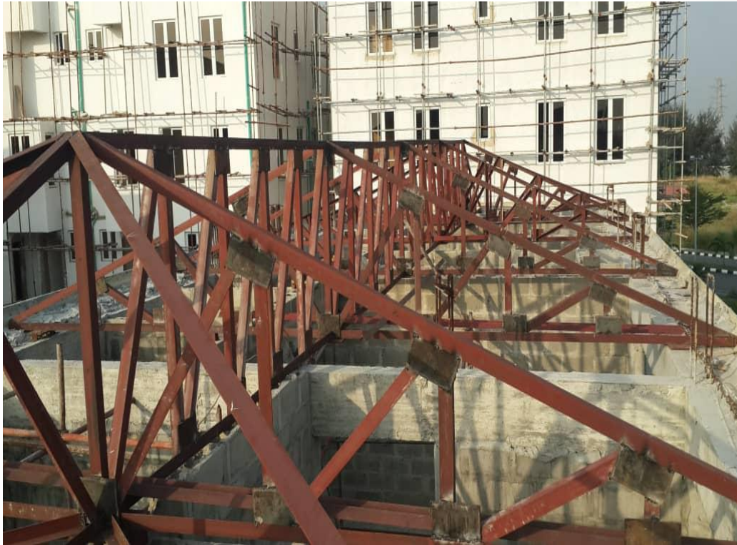
28 – QUOTED STRUCTURAL STEEL FRAMED ROOF AT BANANA ISLAND.
