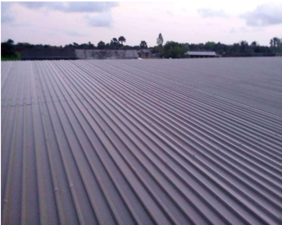
6 - POLYURETHANE FOAM ALUMINIUM ROOFING SHEET, IKEJA GRA.
