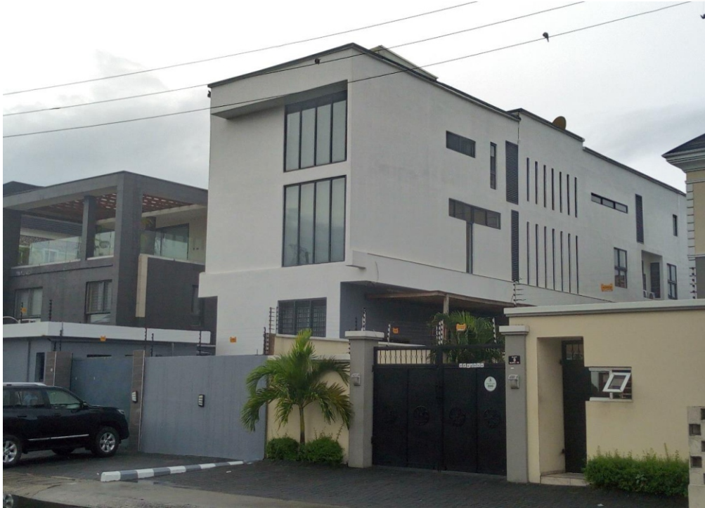
44 - LAMINATED STRUCTURAL CURTAIN WALL IN LEKKI.
