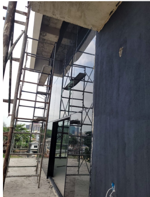
CONCEALED GRID ALUMINIUM FRAMED GLAZED CURTAIN WALL AT MEKUNWEN CLOSE, IKOYI.
