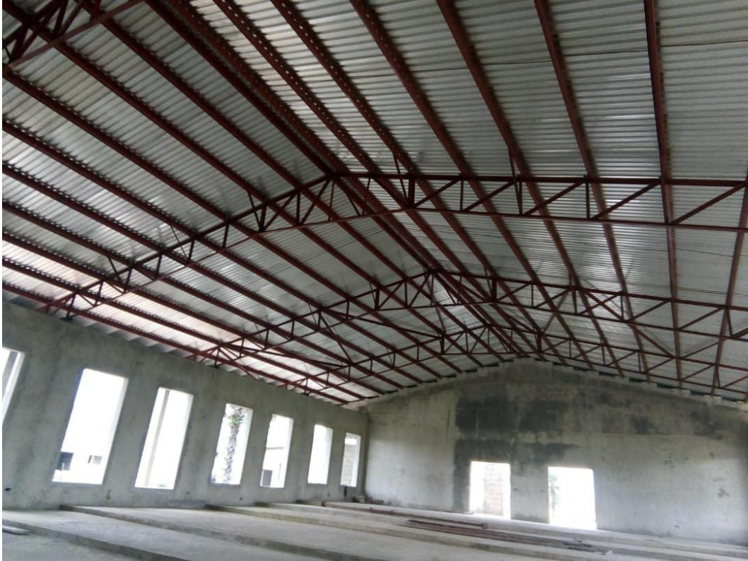
26 – COATED MILD STEEL FRAMED ROOF TRUSS FOR LECTURE HALL AT ILARO.
