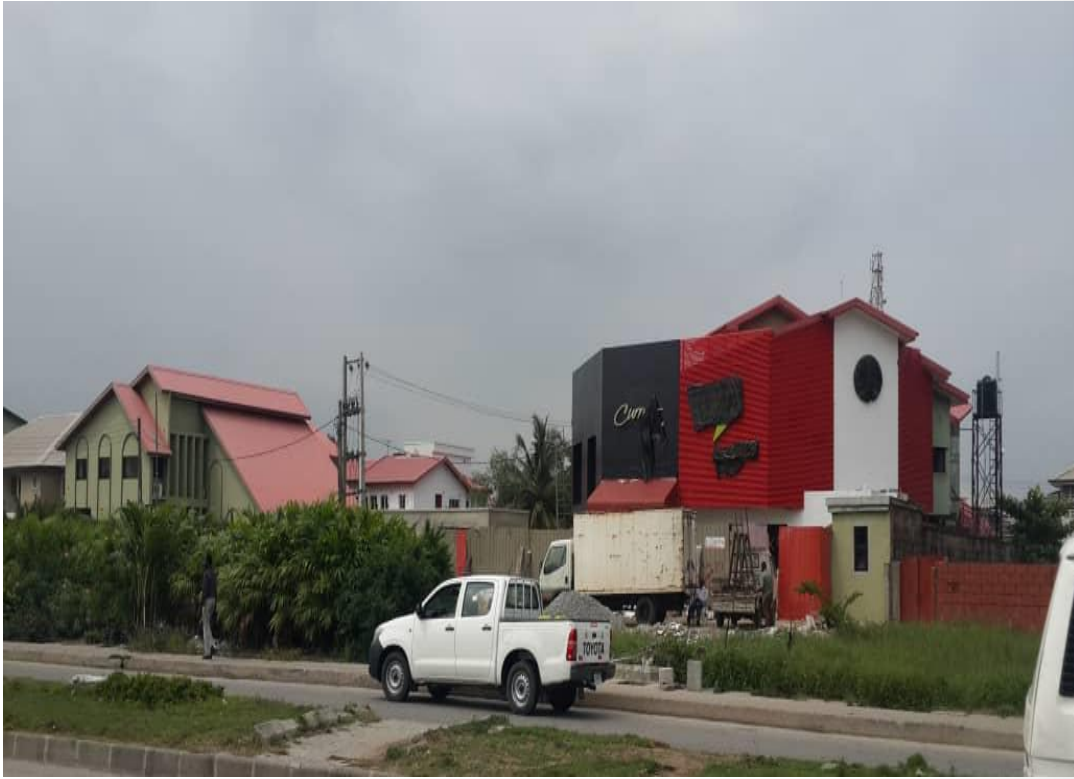
40 – ALUCOBOND CLADDING/ALUMINIUM SUN SCREEN FOR KOBIS OUTLET, LEKKI.
