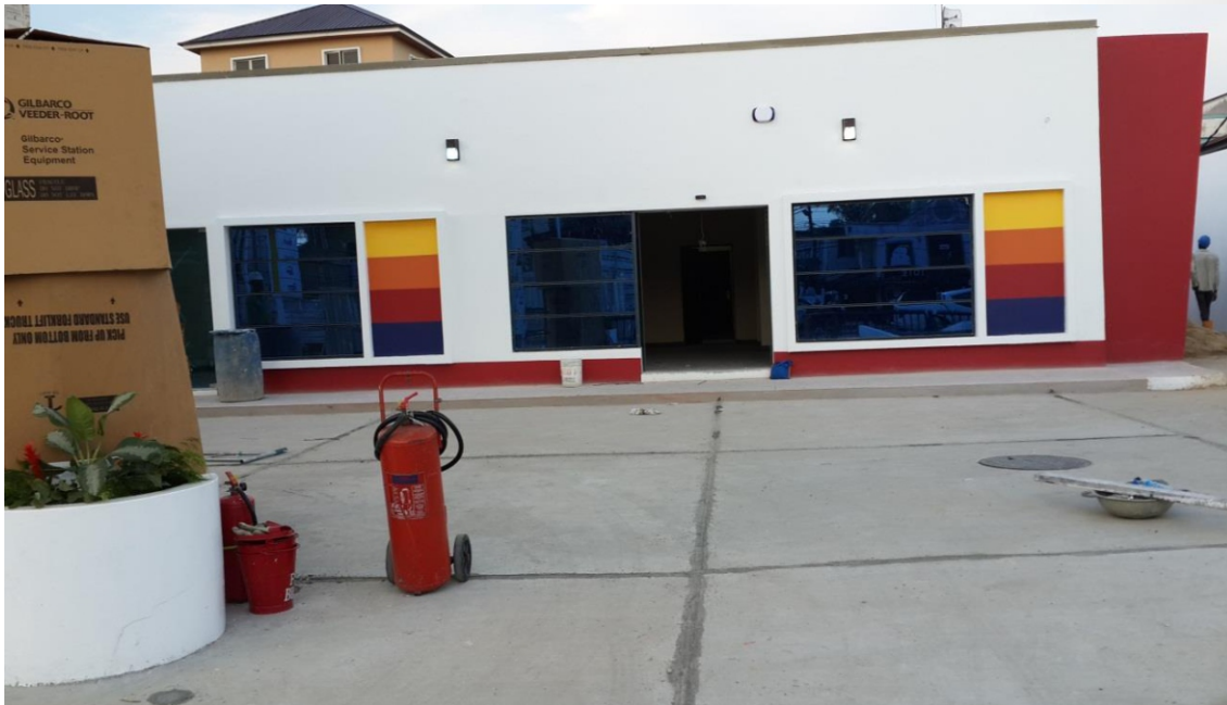
ALUMINIUM CURTAIN WALLS, WINDOWS AND FRAMELESS GLASS DOORS FOR OANDO OUTLET IN AWOLOWO RD, IKOYI, LAGOS.
