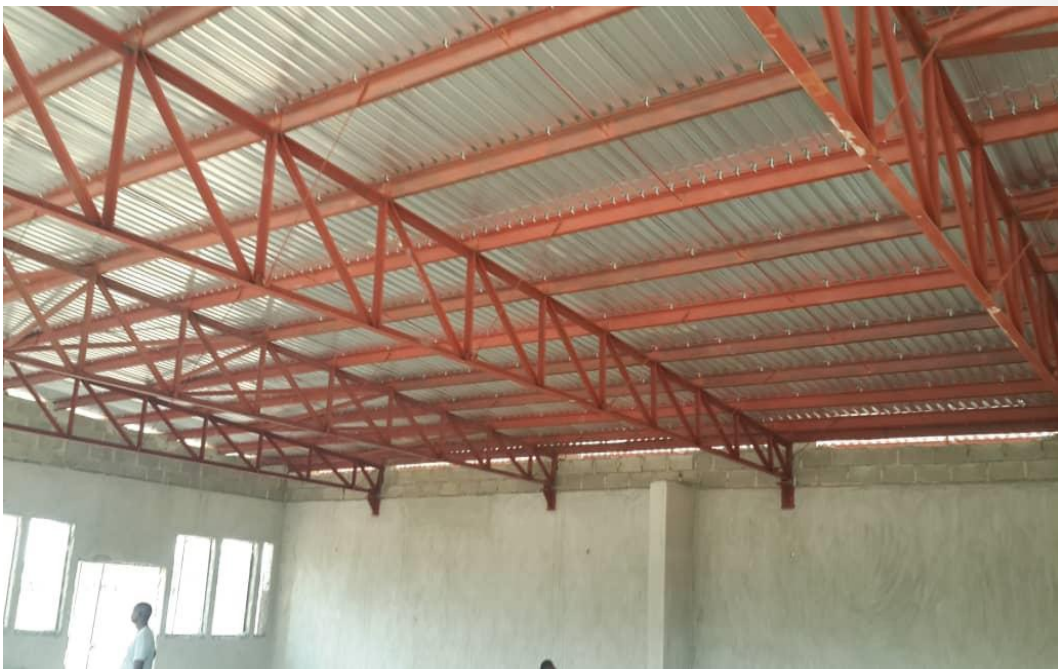
27 – COATED MILD STEEL FRAMED ROOF TRUSS FOR LECTURE HALL AT ILARO.
