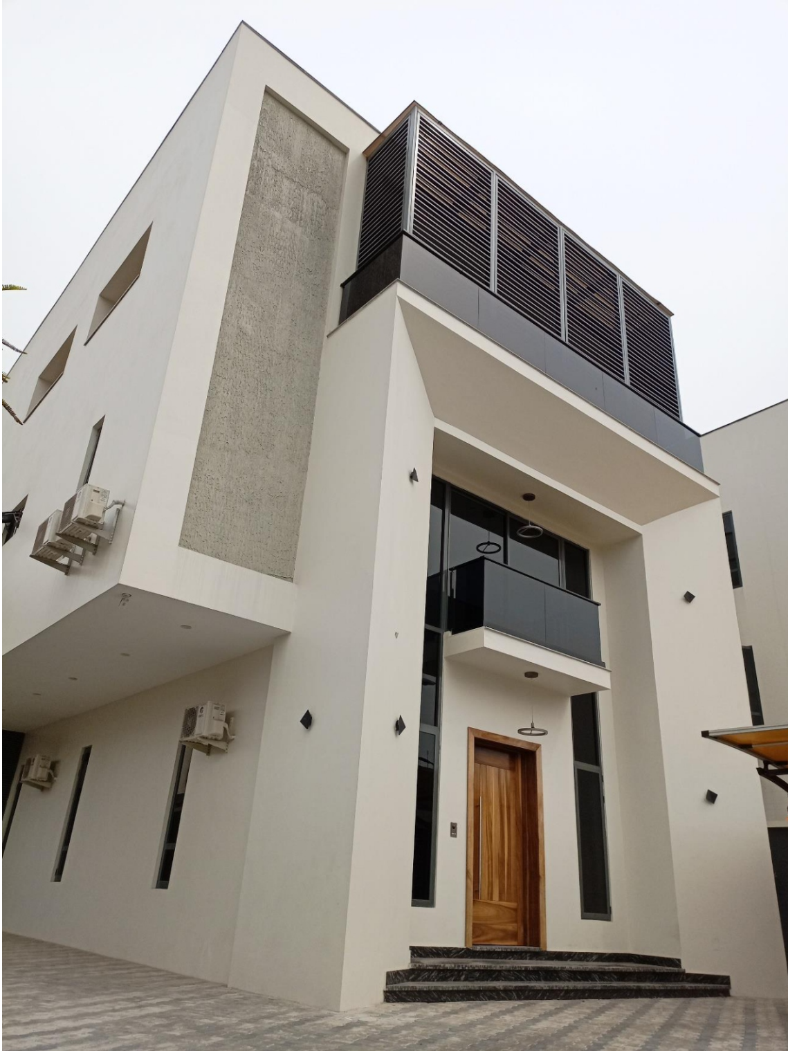
2 – ALUMINIUM LOUVRE SUN SCREEN AT LEKKI PHASE.
