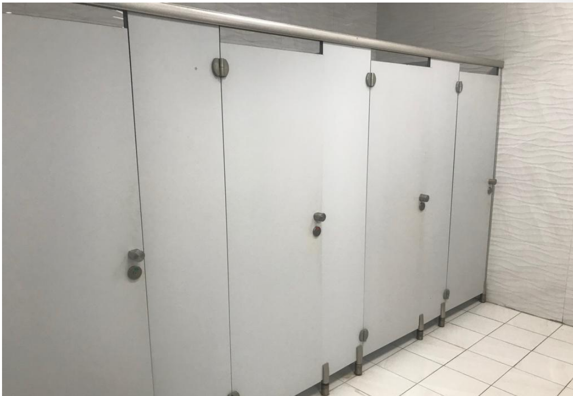
8 – HIGH PRESSURE LAMINATE (HPL) TOILET CUBICLES.
