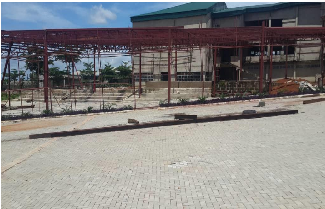
29 – QUOTED STRUCTURAL STEEL ROOF FRAME IN IKORODU.
