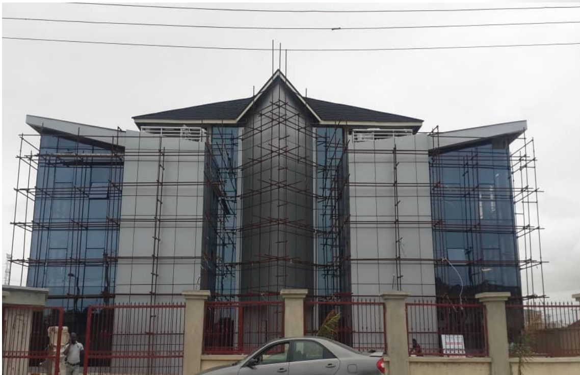
DOUBLE GLAZED STRUCTURAL CURTAIN WALL WITH ALUCOBOND CLADDING.
