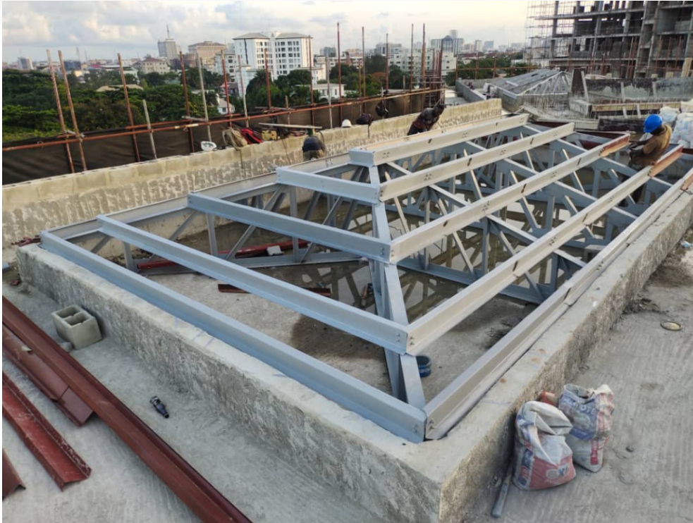
EPOXY COATED STRUCTURAL STEEL FRAMED ROOF STRUCTURE AT ST. SAVIOURS SCHOOL, IKOYI.
