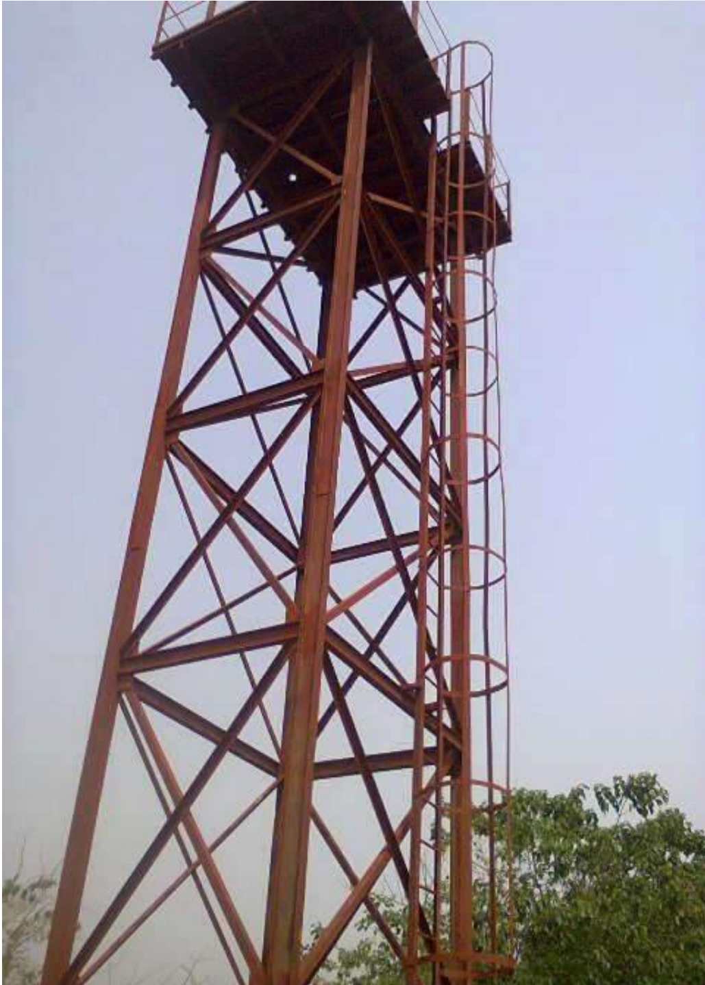
3 – ELEVATED COATED METAL WATER TANK SCAFFOLD.
