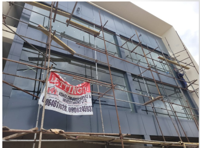
ALUBOND CLADDING/FRAMELESS GLASS SHOPFRONT AT CMD RD, IKOSI- KETU , LAGOS.
