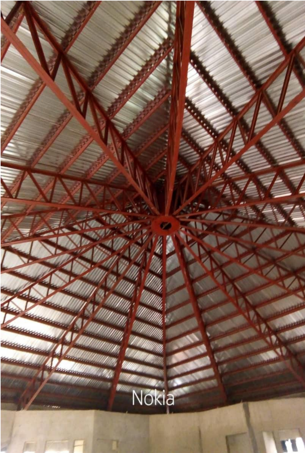
30 – QUOTED STRUCTURAL STEEL ROOF FRAME IN IKEJA.
