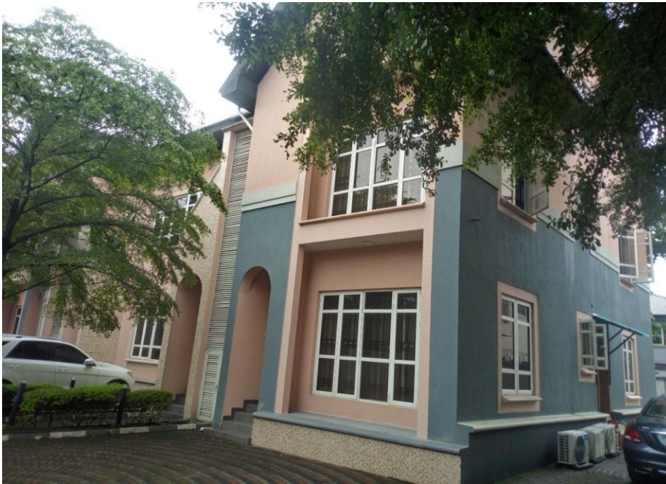
51- ALUMINIUM WINDOWS & DOORS FOR RESIDENCE IN LEKKI.
